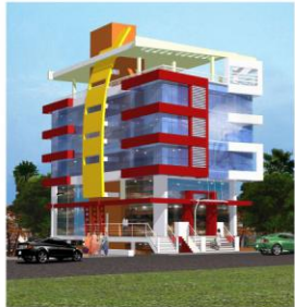
Commercial Complex Kottara Chowki Mangalore
